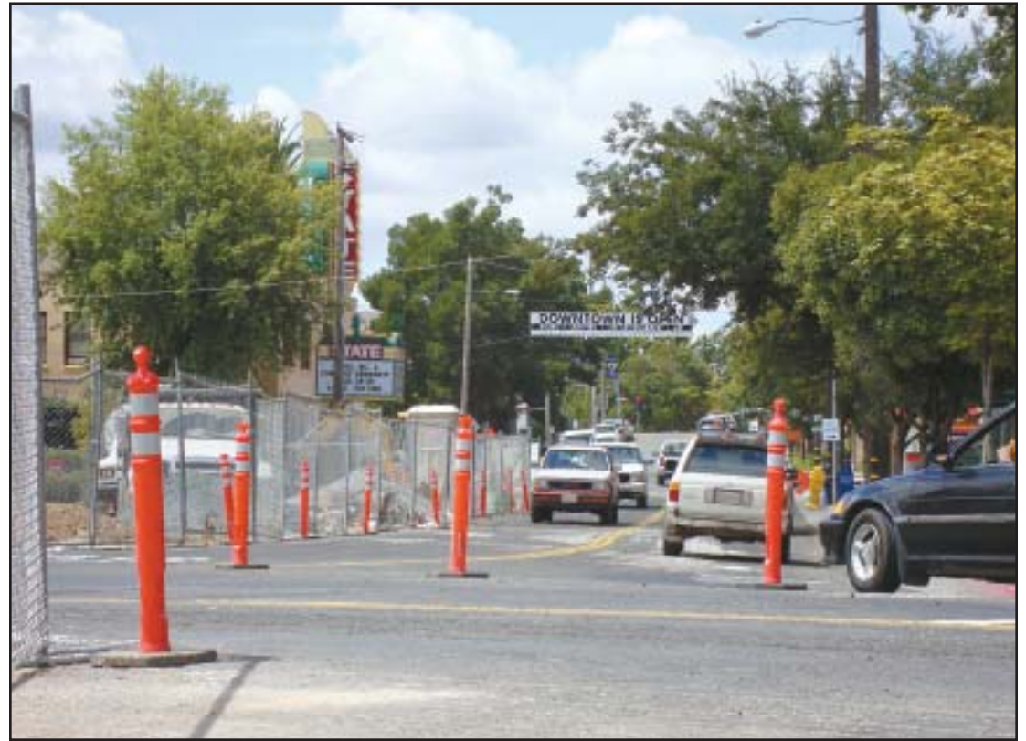
Streetscape construction gets underway at the intersection of Lincoln Way and High Street in Auburn. Photo credit Cheri March.
